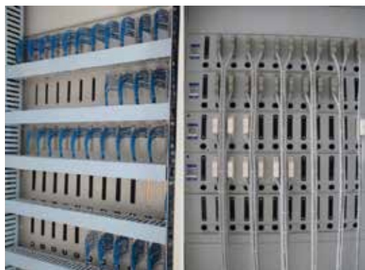
(a)传统接口柜 (b)工厂化接口柜 (a) Traditional interface cabinet (b) Factory fabricated interface cabinet
